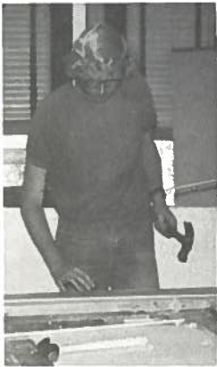
Harry Westerhof helps to ready the building
