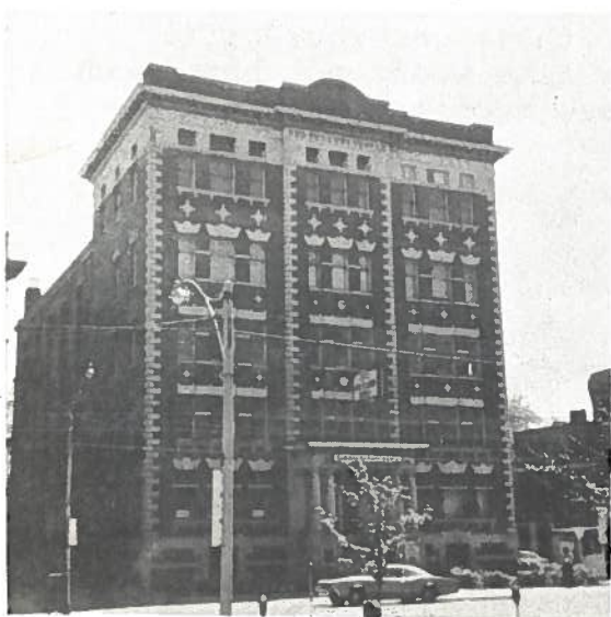
Three Quarter View of the New ICS Building
